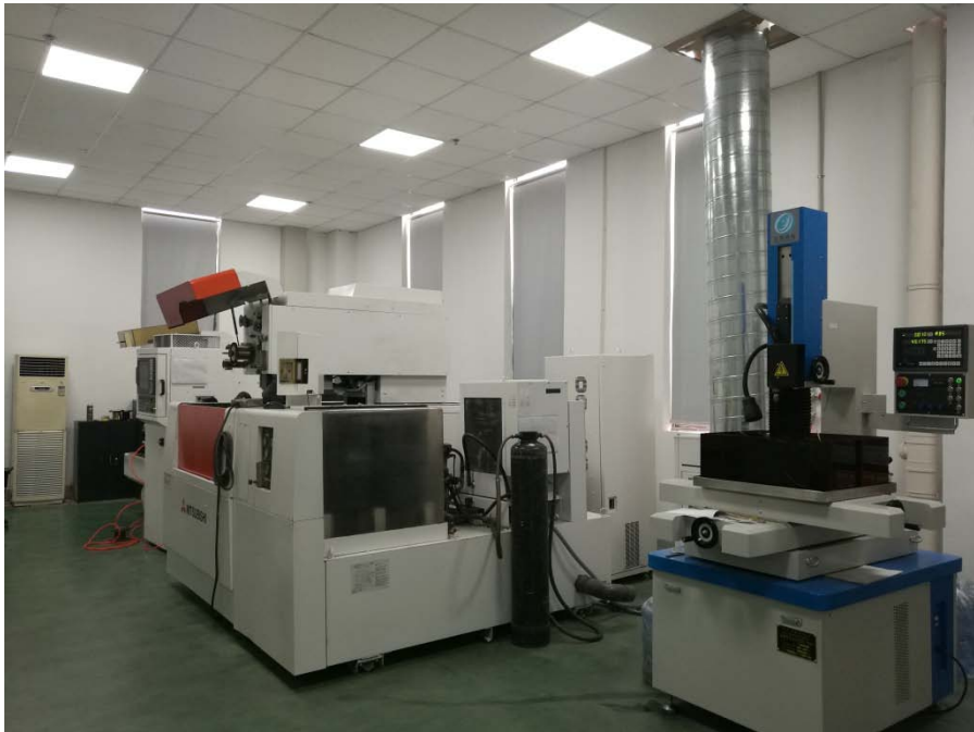
Wire Electrical Discharge Room
